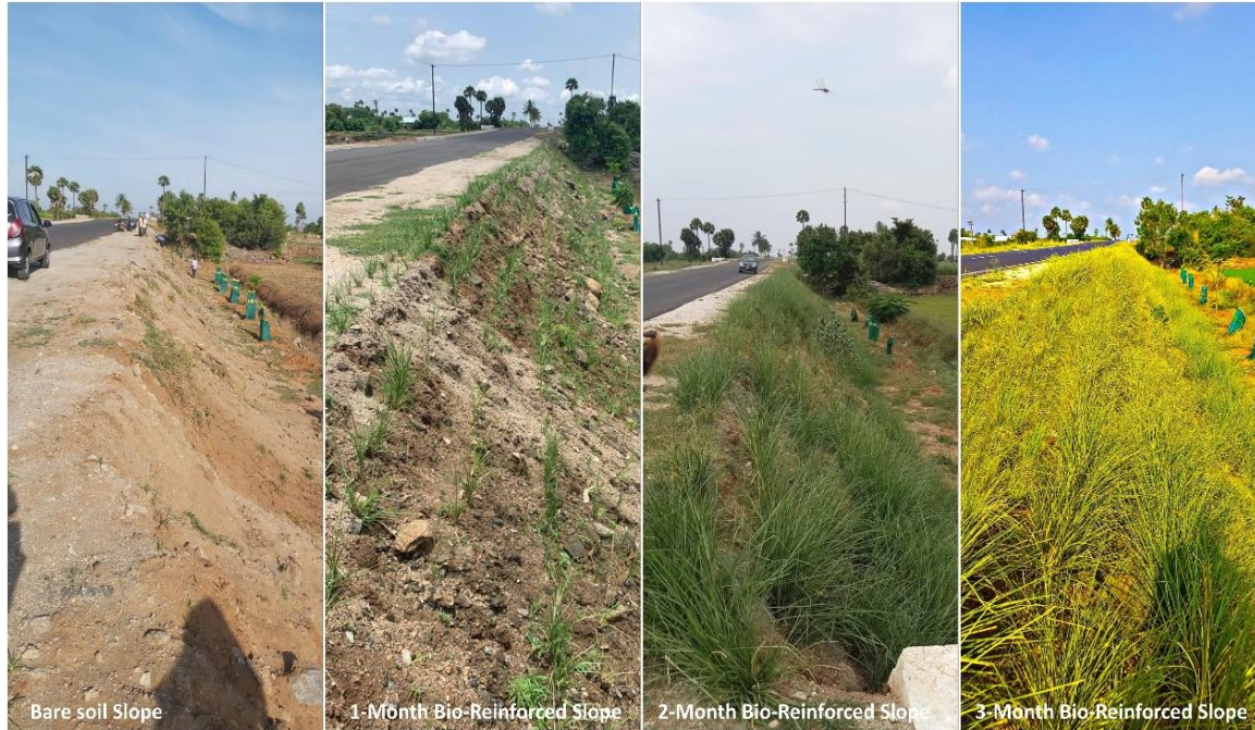
Fig. 1 Field conditions of the reference Rasipuram road embankment, transitioning from bare soil to 3-month-old bio-reinforced slope
