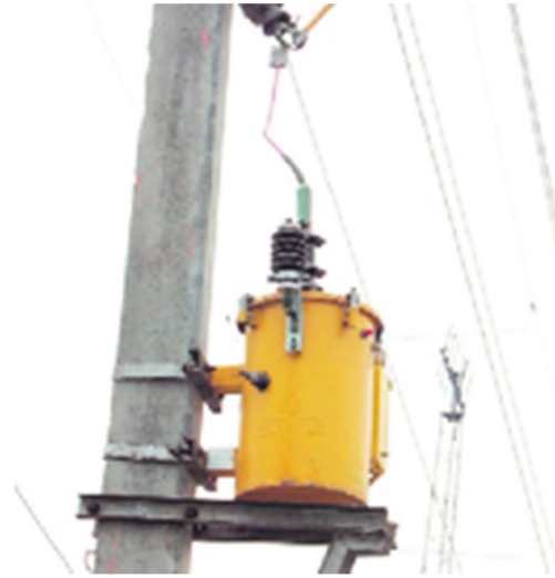
Fig III: single phase HVDS
