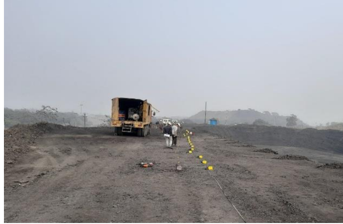
Fig. 3 Installation of ATOM geophones for ISRT
