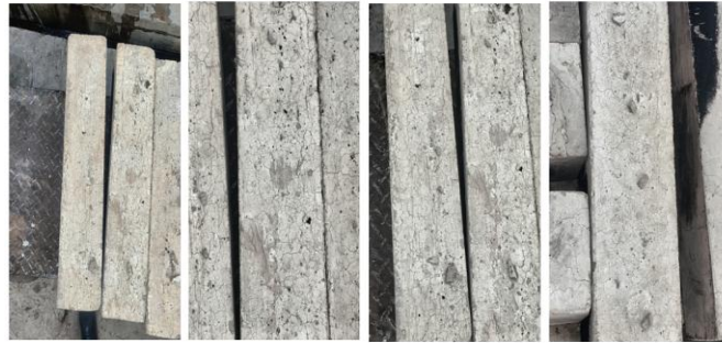
Fig. 3 Specimen after fire exposure at different temperatures (visible cracks)
